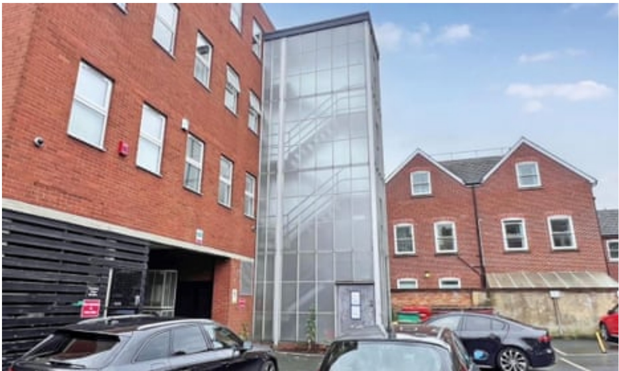
The stairwell in Twickenham
